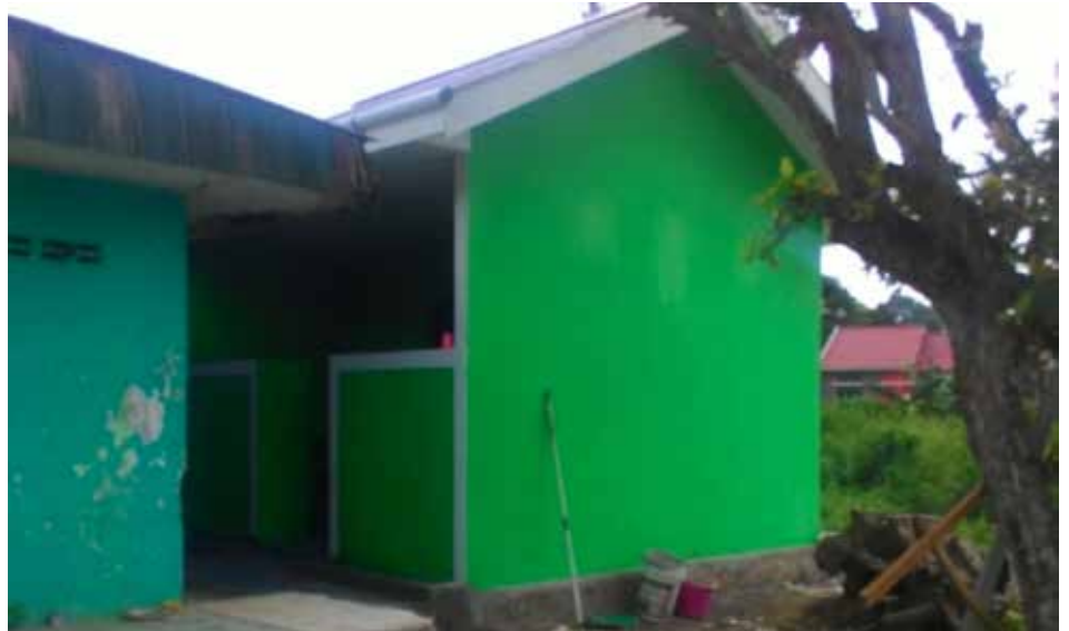
The new shower and toilet block abutting the older facility
