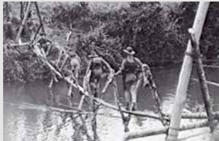
V-shaped bridge built by a pioneer platoon for a creek crossing on the Kokoda Track
