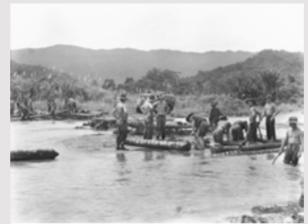
Typical work and conditions for the Pioneer Platoon in the Ramu-Markham Valley
