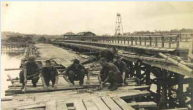
Repairs being carried out on the Manggar River Bridge. Thorpe's Tower at rear.
